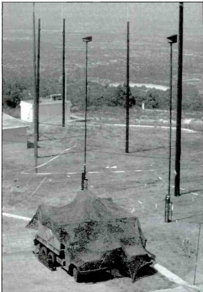
← A mountain-top U.S. Army radio facility in California. (Army photo)
