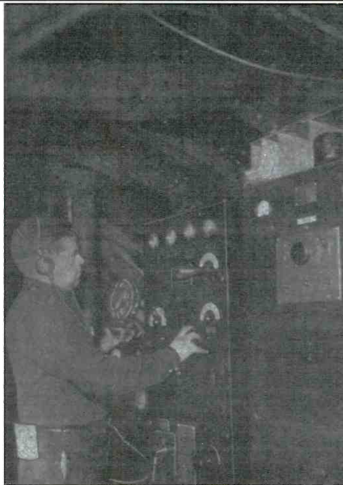
The 200-watt G.E. transmitter aboard the research submarine, Nautilus .
