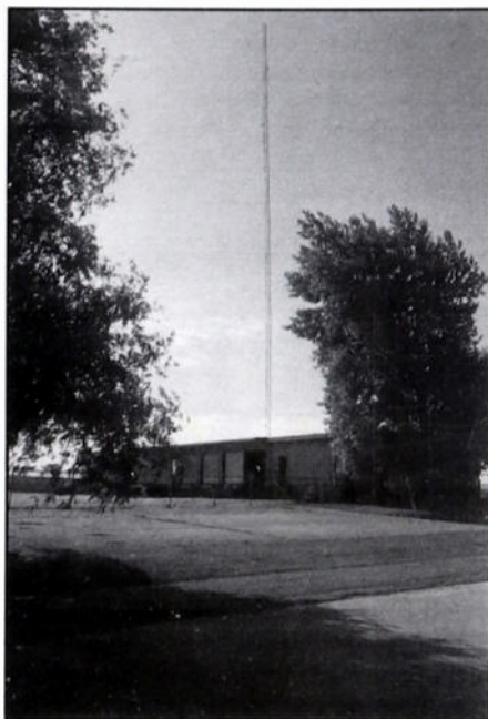
This tower is located at a small trucking terminal in West Burlington, Iowa. The tower is used to maintain contact with on-the-highway trucks. To find highway trucks in your area, search between 43.86 and 44.42, 159.495 and 160.200, and 452.375 and 452.875. (Photo by Chuck Gysi, N2DUP)
