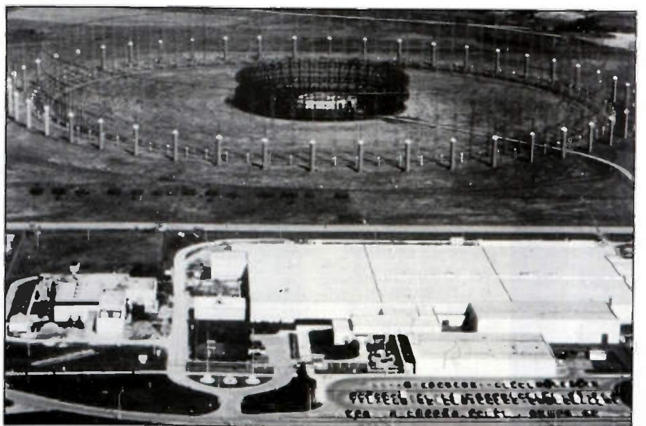
An anonymous contributor sent in this photo of the now-closed U.S. Army Field Station at Augsburg, Germany. It was the largest SIGINT site in the free world. The antenna, an AN-FLR/9, was located on an old Nazi airfield.
