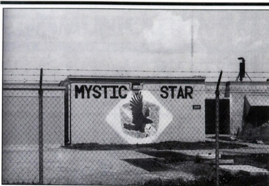
These photos of antenna installations at Scott AFB, IL, were provided by reader Dennis J. Capriglione, MO.
