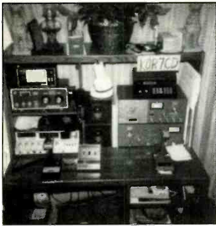
This attractive installation is owned by Ron Dowdy, 7-OT-827, SSB Network member SSB-827D, and Registered Monitor KOR7CD. Ron is from Myrtle Creek, Ore.
