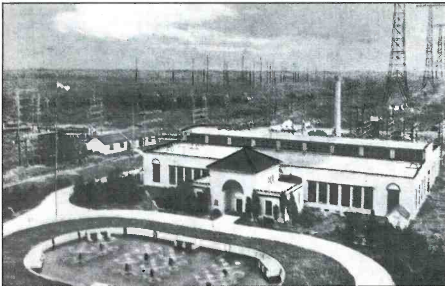
A general view of RCA's Radio Central in the late 1930's.
