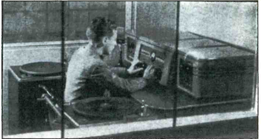
A control room at CKCK in 1938. In order to assure freedom from vibrations, it was a "room within a room." The inner room was supported on thousands of springs.
