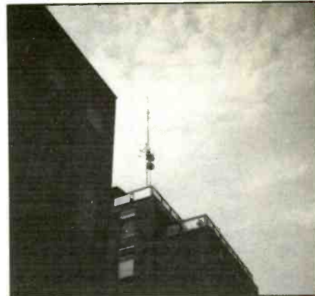
Another tower in Ravenna. Both towers were within a few blocks of the Poste E Telecomunicazzion building at Piazza Garibaldi. Photo courtesy of R.C. Watts, KY.
