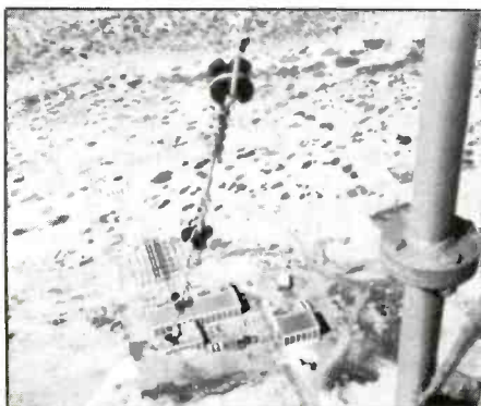
A flying flamingo's eye view of the TWR/Bonaire transmitter and diesel generator buildings as they appeared in 1964 from near the top of the station's 760 ft. medium-wave tower.
