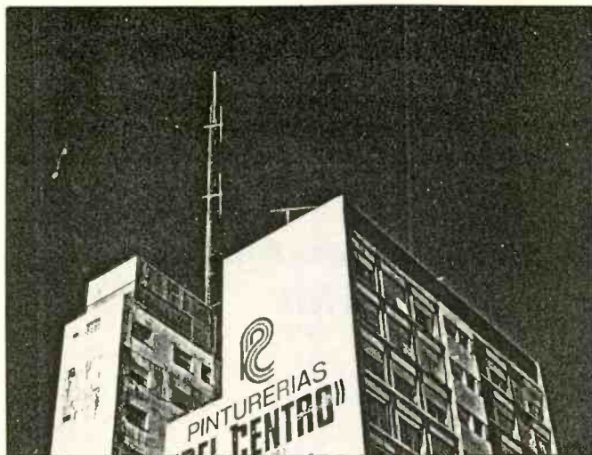
"Radio Llamada" (Radio Call) is the name of a pager in Mar del Plata, Argentina. Operating on 35.22 MHz with 500 watts into a collinear antenna, it has been reported by listeners throughout the world.
