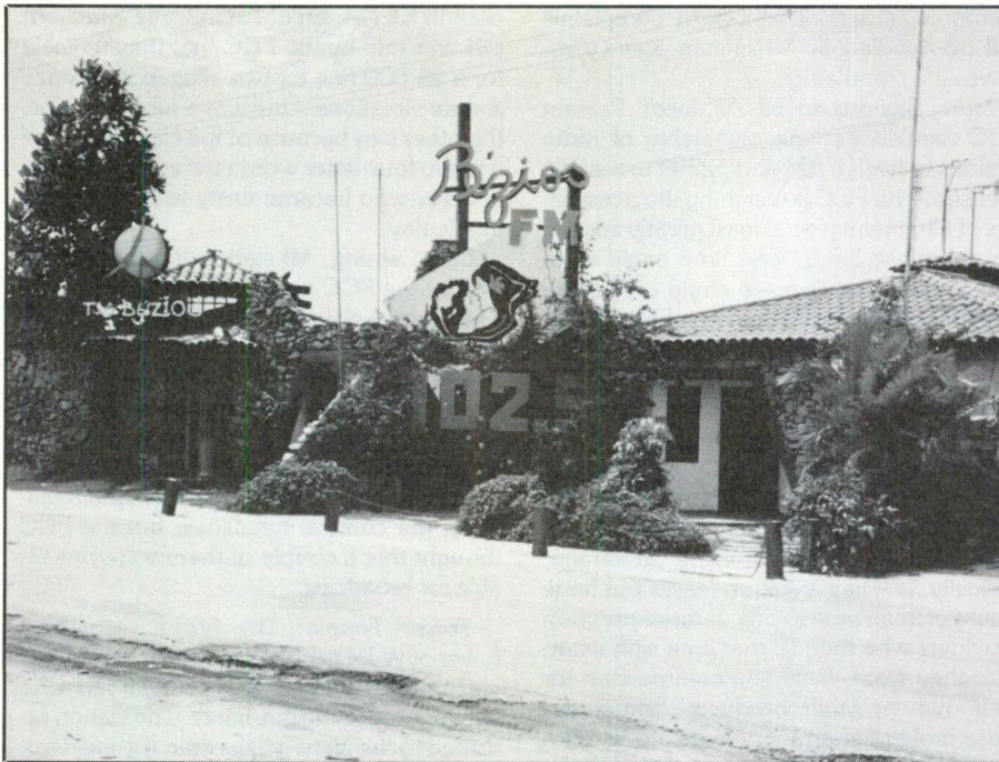
This exotic building in the Brazilian resort town of Buzios houses FM 102.5 and also a UHF-TV station. (Courtesy Helio Soares, Brazil.)
