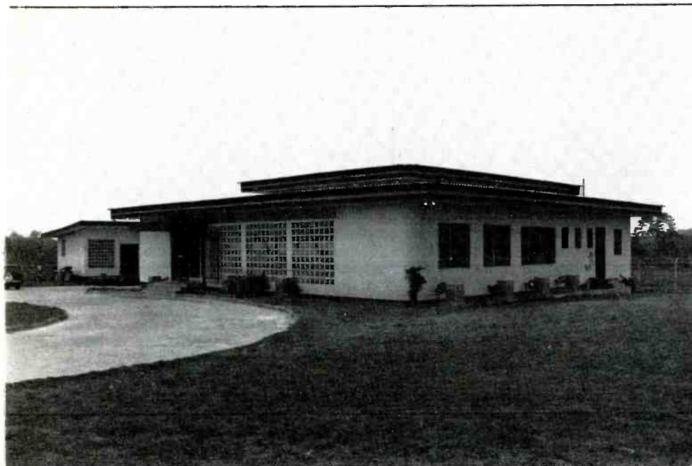
Station ELRG in Gbarnga. Offices, studios and transmitter are housed in a single building. The generator building is on the left.
