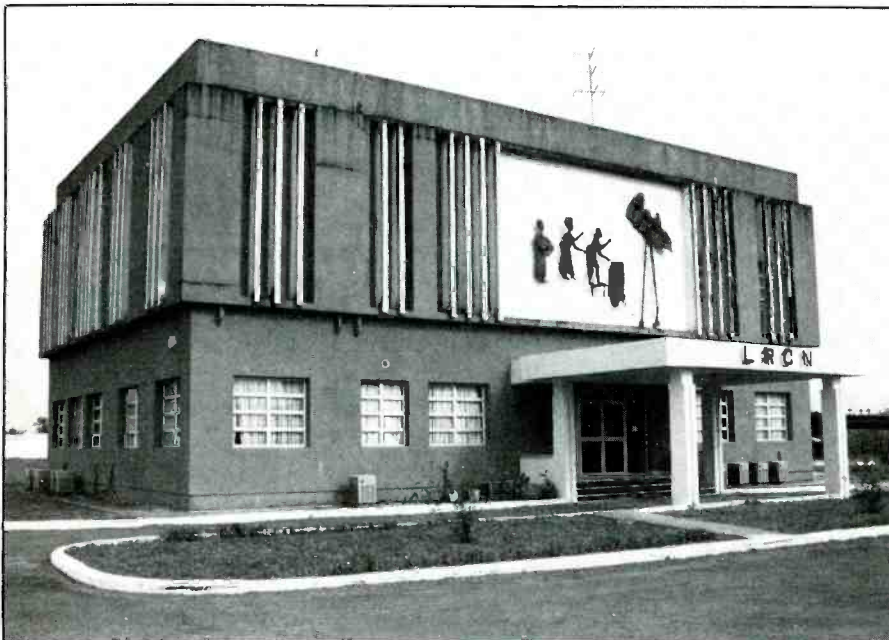
LRCN headquarters in Monrovia, scene of a battle between Government of Liberia and rebel soldiers in a 1985 coup attempt. The antennas on the roof are part of the independent sideband (ISB) studio-transmitter link.
