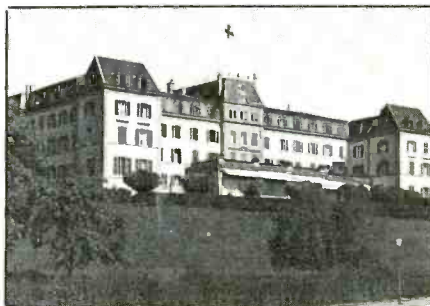
RCBS studios are in the ICRC's headquarters building in Geneva, Switzerland.
