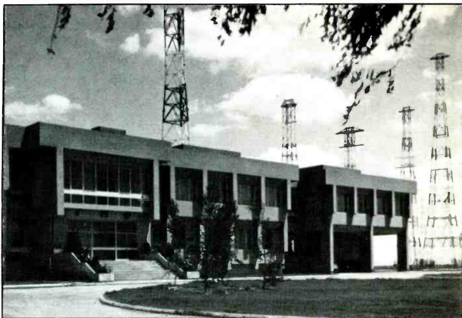
The Radio Nacional Espana transmitter site at Noblejas, Spain.
