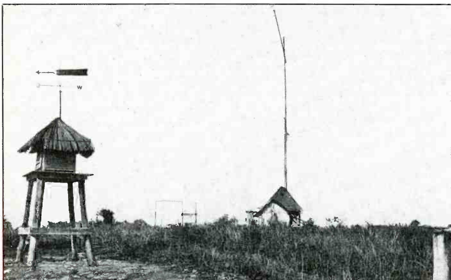
Doesn't look like much, but the shack with the mast in the center of this photo was an early coastal telegraph station at Malabang in the Philippines.
