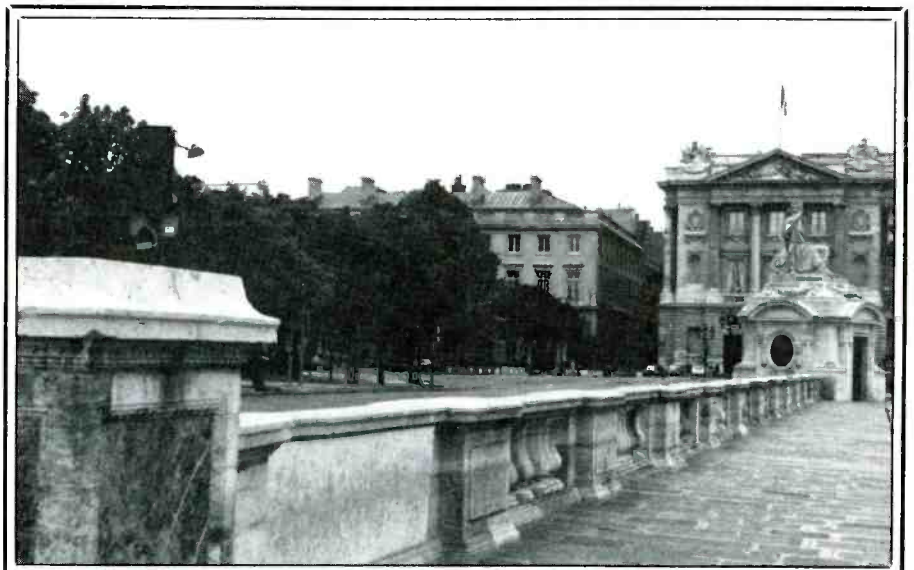
View of the American Embassy, Paris (center), with its antenna farm atop the roof. (Photo by Robert Margolis.)
