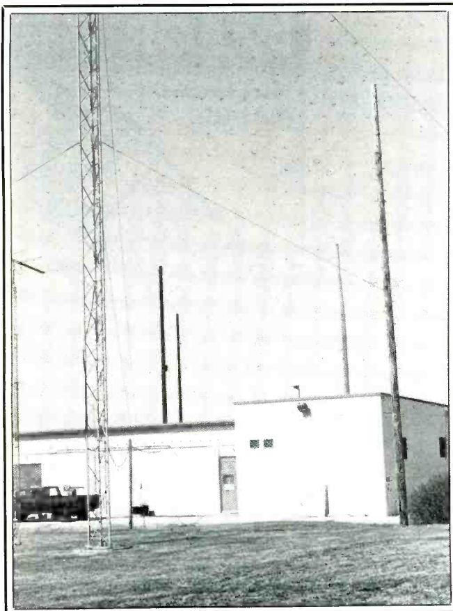
Exterior view of U.S. Air Force Military Affiliate Radio Station, Scott AFB, Ill. (U.S. Air Force photo by Sgt. Ron Reed)
