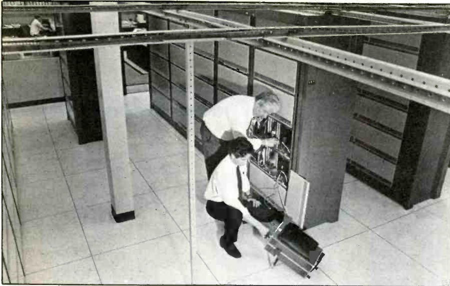
Los Angeles Cellular Telephone Company became the first cellular carrier to activate a second digital switch. The dual switch system allows L. A. Cellular to double its call processing capacity to accommodate an increasing demand for cellular service in Southern California.
