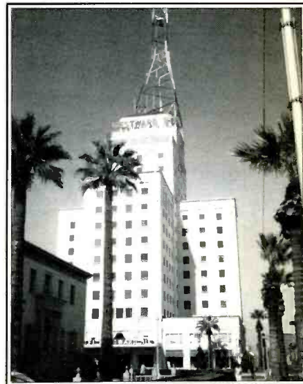
The old "Westward Ho" Hotel, in Phoenix, AZ, at one time might have carried an old AM station. Now, it supports many utility and public service VHF and UHF antennas.
