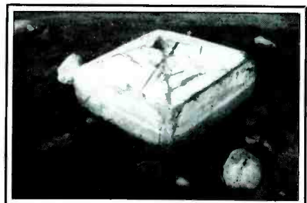
All that presently remains of the old Brant Rock station is this concrete footing reputed to be the base of the tower. Most likely it is actually an anchor for one of the guy wires. (Courtesy Robert Fraser.)
