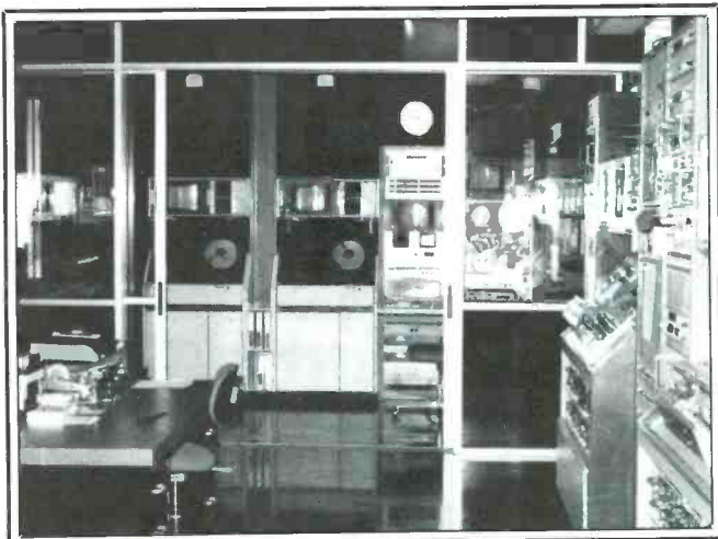
It's hard to visualize just how large a metro TV station is. These two photos show about half of the video tape area at WBAL-TV. If you look beyond the desk in the center of the left photo you see the window and doors leading to the control room seen in the film Diner. The big brutes with the ovals in the center (right photo) are TV cartridge machines. To the right are many cassette machines used, among other duties, to play the cut-ins on newscasts. The station has about 20 tape machines in this area.
