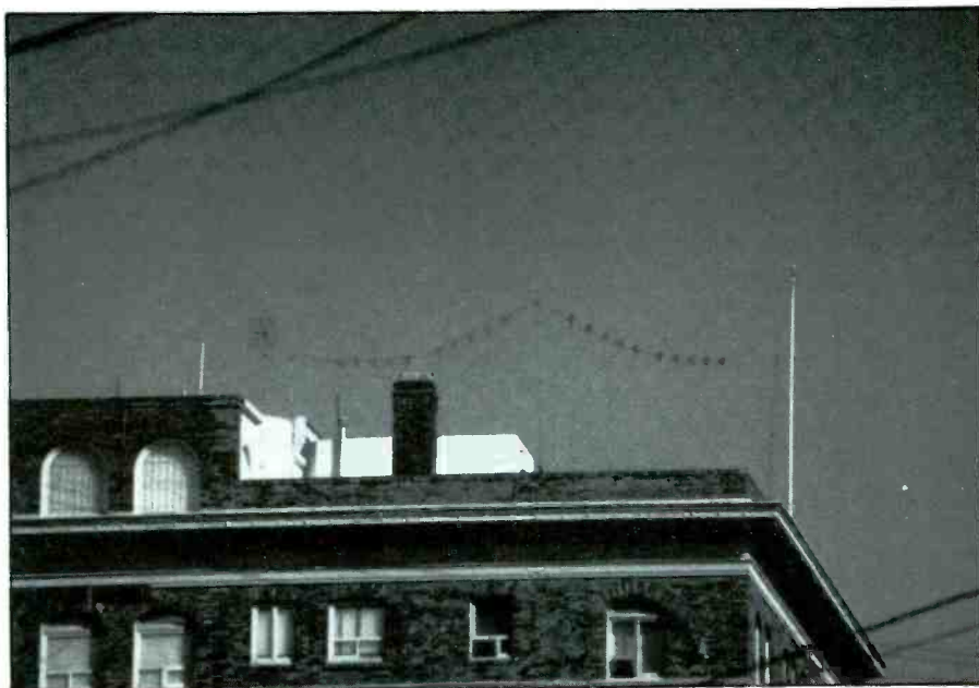
In December of 1982, without warning nor building permit, antennas began appearing on the roof of the Soviet Consulate in San Francisco. This view is from Baker Street. (Photo by Bill Schworger, KA6TOL)
