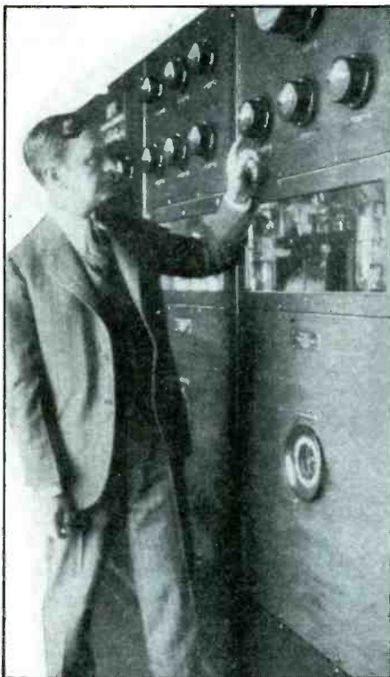
Reading the meters on the 5 kW transmitter used by KFI. This photo was taken in early 1926. The meter reader is none other than Sol Lesser, a well-known motion picture producer of the era.
