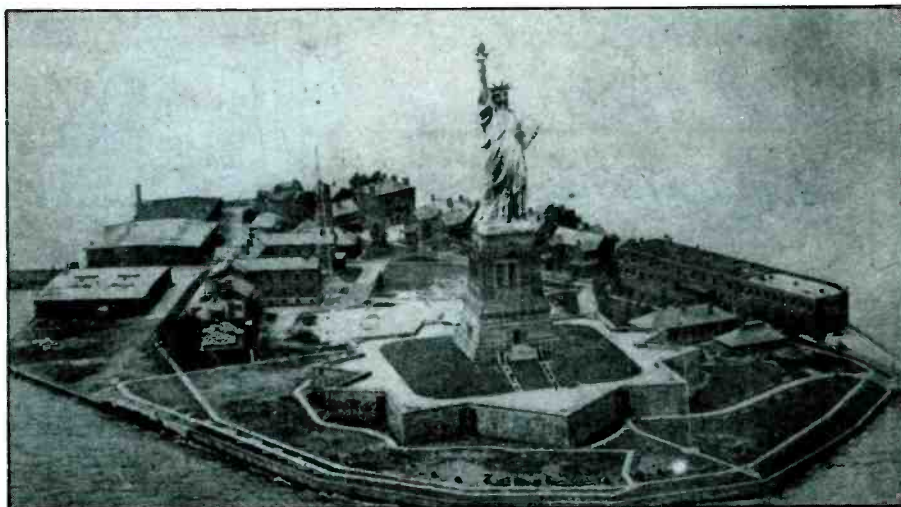
In this aerial view of Bedloes Island in 1922, two radio towers are on the scene. One is to the left-rear of the Statue of Liberty, midway between the Statue and the island's shore. The other tower is located at the upper left shoreline and is just about impossible to see (even on the original photo).
