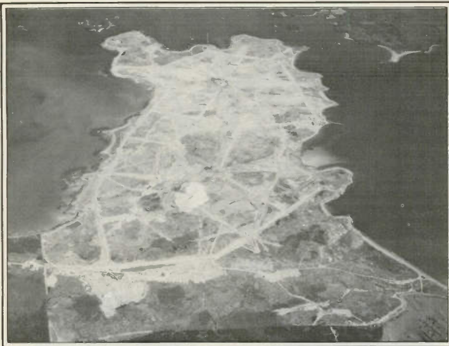
The antenna system of NAA covers many acres of land. (Photo courtesy U.S. Navy)
