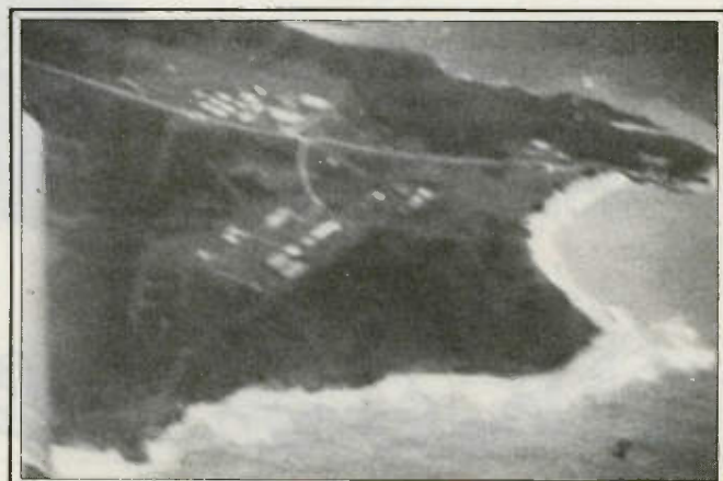
Aerial view of Swan showing the western end of the island. The RA compound is at the top of the photo. Federal compound is towards the bottom.
