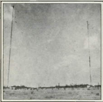
The antenna system at Radio Americas.
