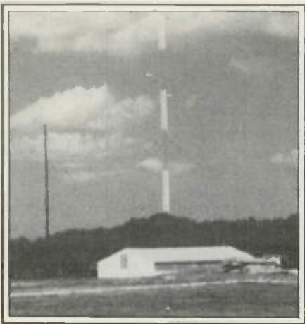
At the federal compound, the FAA's radio range tower looms high above the dense but low foliage.
