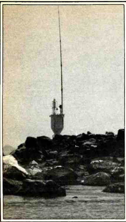
The 200 to 400 kHz band swarms with radiobeacons, many even transmit weather information. The AIR-8 can receive these stations. This photo of a low frequency marine radiobeacon was taken by Michael Mideke.
