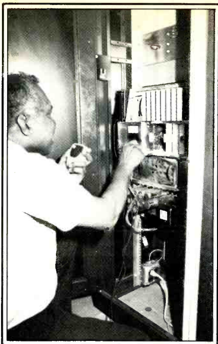
Bruno Johnson is shown here monitoring the emergency control stations standby, in the event of a main system failure.
