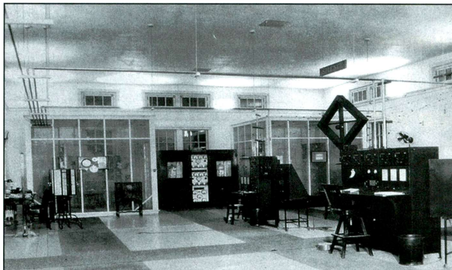
Photo B. Here’s a view inside the Monitoring Room on the north side of the building as it appeared in 1932. This is the same room KDØHKD saw on his tour of the facility in the early 1980s. Equipment included primary and secondary standards and an all-wave receiver. (U.S. Government photograph, courtesy of KDØHKD)
