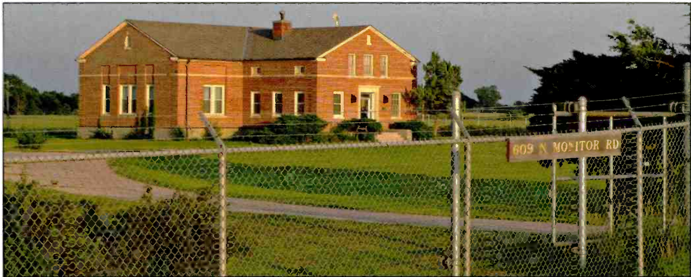
Photo E. Here's a view of the station from the northwest, showing the classic street address plaque. To the communications aficionado, the name of the road is a dead giveaway to the building's use. (Courtesy of Creative Commons CC0 1.0 Universal Public Domain Dedication)
