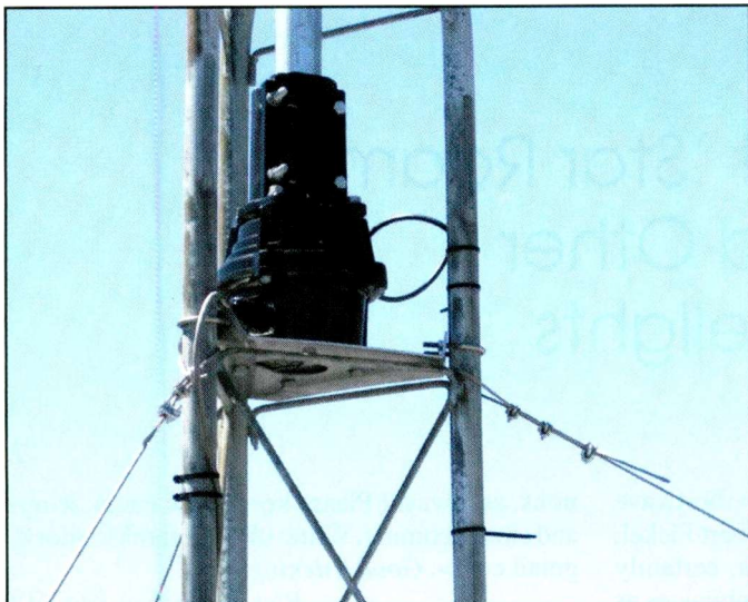
Photo B. When it comes to bang for the buck in medium-duty antenna rotators, Yaesu's G-800SA is hard to beat. This picture-perfect installation is at W7MRE, The American Museum of Radio and Electricity in Bellingham, Washington. (Courtesy of AE6K)
