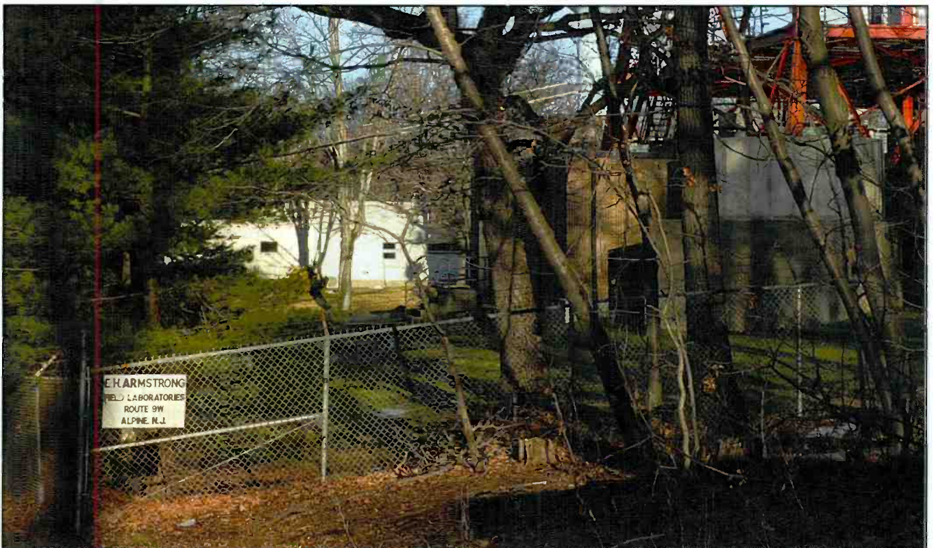
Photo D. The historic Armstrong site remains an active communications facility today, so public access is restricted with the area secured by a barbed wire-topped fence.
