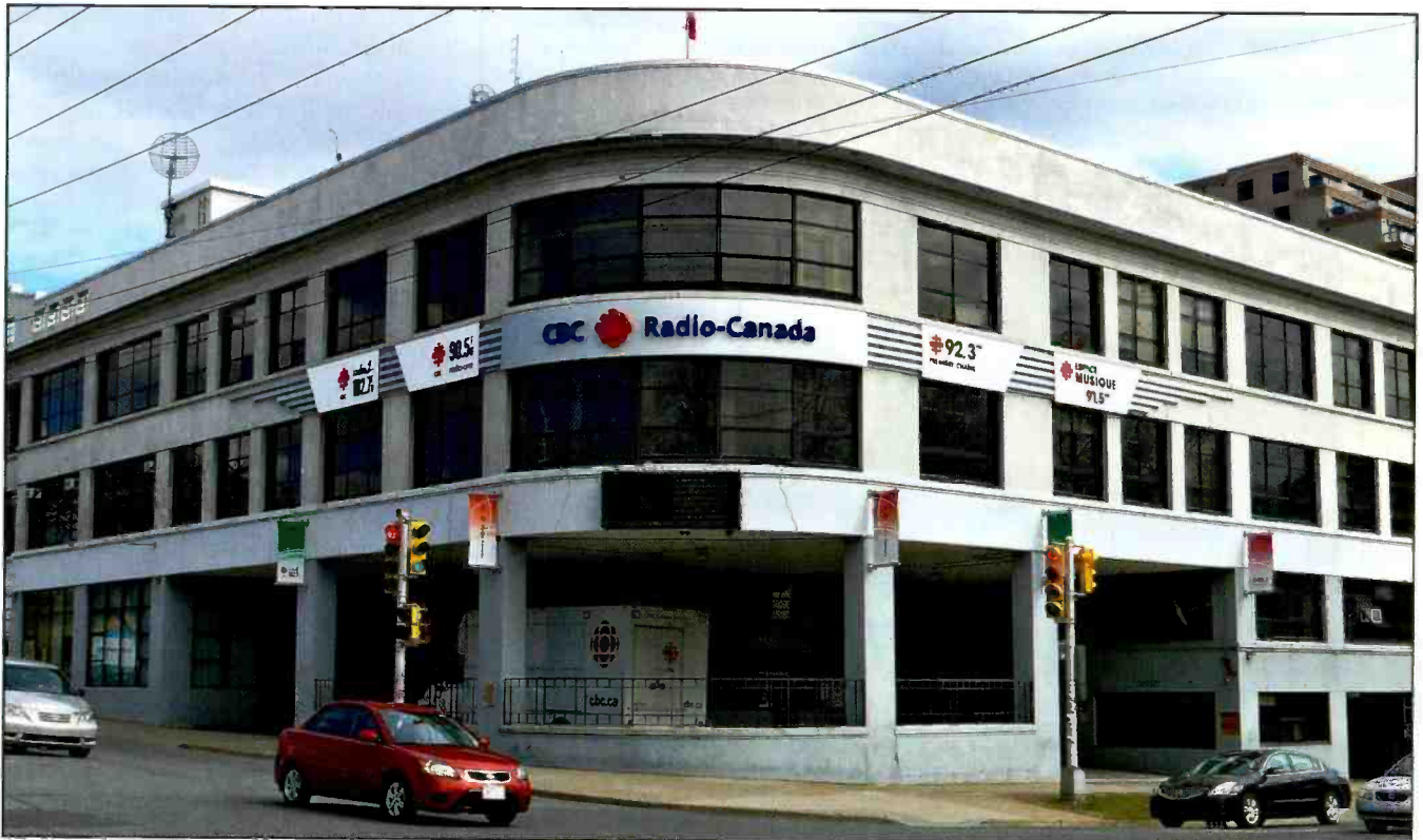
Photo D. In 2010 CBC Radio agreed to sell its building on the corner of Sackville and South Park streets, in Halifax, Nova Scotia, Canada to developers — whose plan was to demolish it in favor of condominiums. Radio operations were moved to an expanded CBC Television building on Bell Road. (Courtesy of Halifax, Nova Scotia, Canada via Wikimedia Commons)
