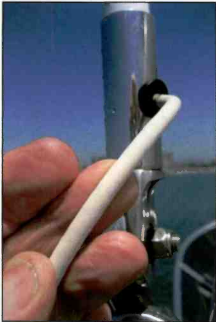
Photo F. Carefully inspect VHF antenna coax leads. If you spot cracks in the jacket, the antenna system needs to be replaced.
