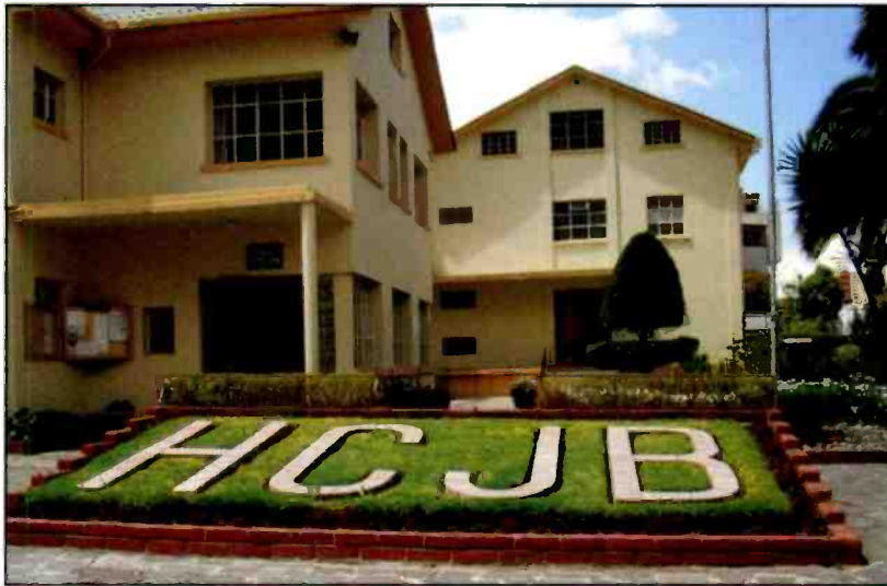
Photo A. This 2007 picture of HCJB is no doubt a far cry from how things appeared 80 years ago when the missionary station went on the air for the first time from Quito, Ecuador — running 200 watts. (Courtesy of Mschaa via Wikimedia Commons)
