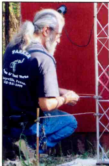
Rich Parker, Pennsburg, PA, works on the ground system at his recently constructed separate shack.
