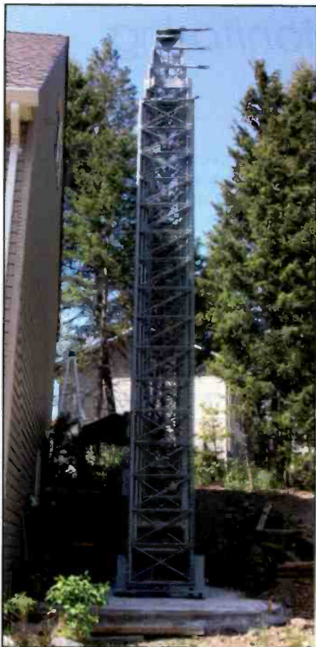
Photo C. When it's time to hunker down , the 90-foot tower at VEPC1CQ can be compacted to a package that's about the same height as the house it stands beside.
