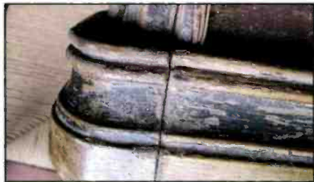
Photo F. Here is the detail of the left column. Mornhinweg suspects it had black dye in most of it, but brown at the sides (left side here). "All of that remains only in the low areas; at the raised areas the finish was totally worn off. Later, someone painted over it all, with yellowish brittle stuff."
