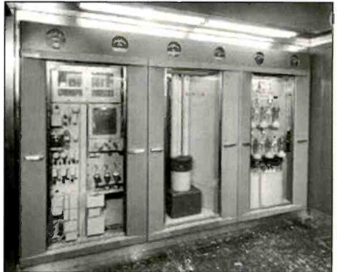
What radio buff wouldn't mind eating off the floor in front of this squeaky-clean Western Electric 50-kW AM rig? It, and a 455 tower mate, was new to KSL in 1940.
