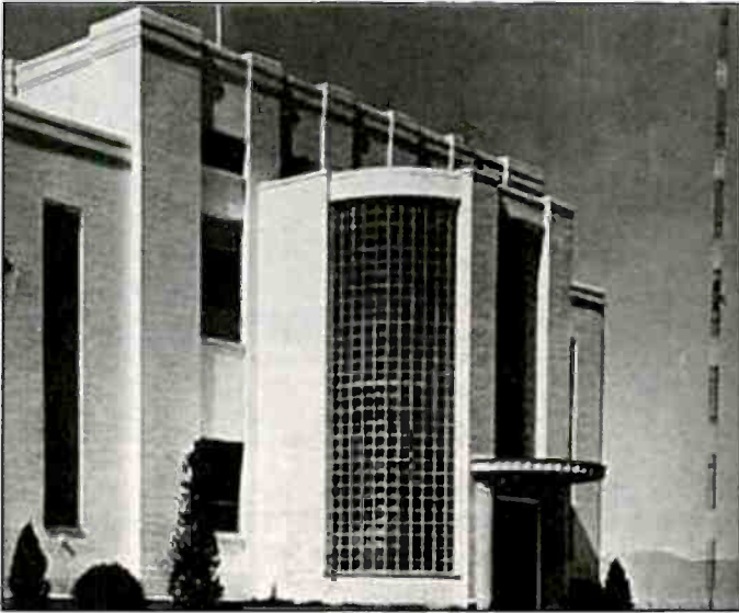
KSL's new (1940) transmitter building in Saltair, Utah, sure can't be called an Xmitter shack. It looks more like a transmitter tabernacle suitable for broadcasts of the Mormon Choir!
