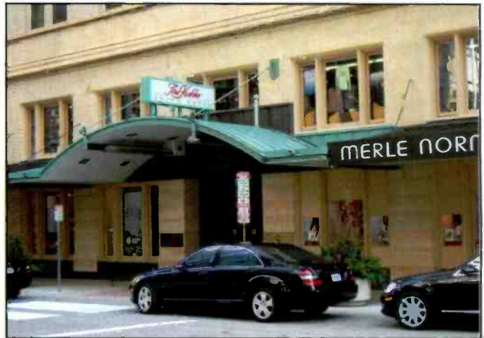
Downtown hotels might use frequencies for maintenance, security, housekeeping, banquet and convention services, and more. This image of the Kahler Hotel, across from the Mayo Clinic in Rochester, Minnesota, shows Mercedes-Benz vehicles that belong to a security detail for Saudi Arabia's King Abdullah bin Abdulaziz, who was visiting Mayo Clinic for a physical. The Kahler uses 461.125 MHz for security and maintenance. (Photo by Chuck Gysi, N2DUP/scancomm.net)
