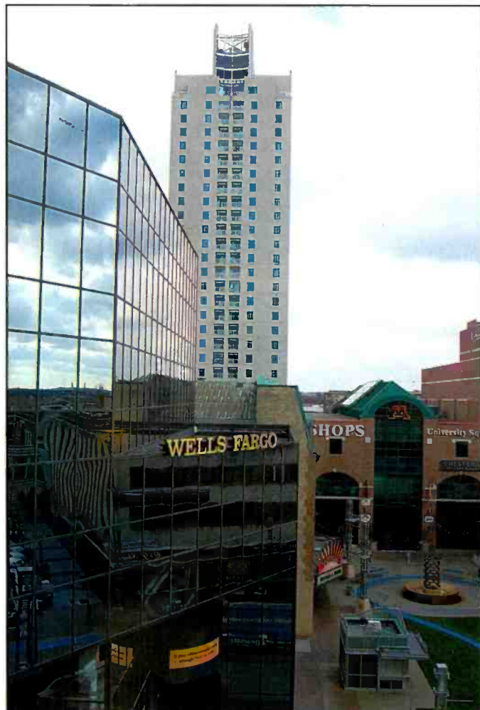
Search business frequencies in downtown areas to find those used in office buildings, retail operations, and other institutions, such as medical facilities. This image shows office buildings, shopping facilities, and a large hotel in downtown Rochester, Minnesota. UHF business frequencies are favored by downtown business users because they bounce around buildings best. (Photo by Chuck Gysi, N2DUP/scancomm.net)
