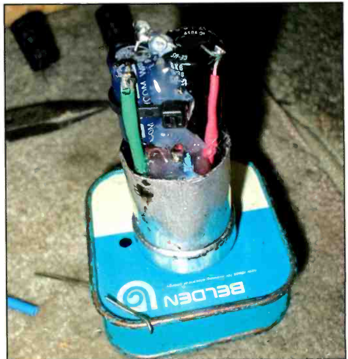
Photo H. Space is tight and all of the available room was needed to house the three replacement caps in this can. Note that heatshrink tubing or insulating "spaghetti" covers any exposed leads. A few dabs of hot glue hold the parts in place.
