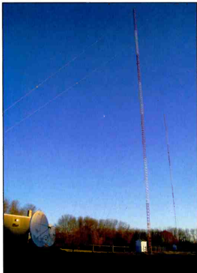
The WDDZ two-tower array of 300-foot, one-sixth wavelength, 550-kHz antennas aimed southeast.
