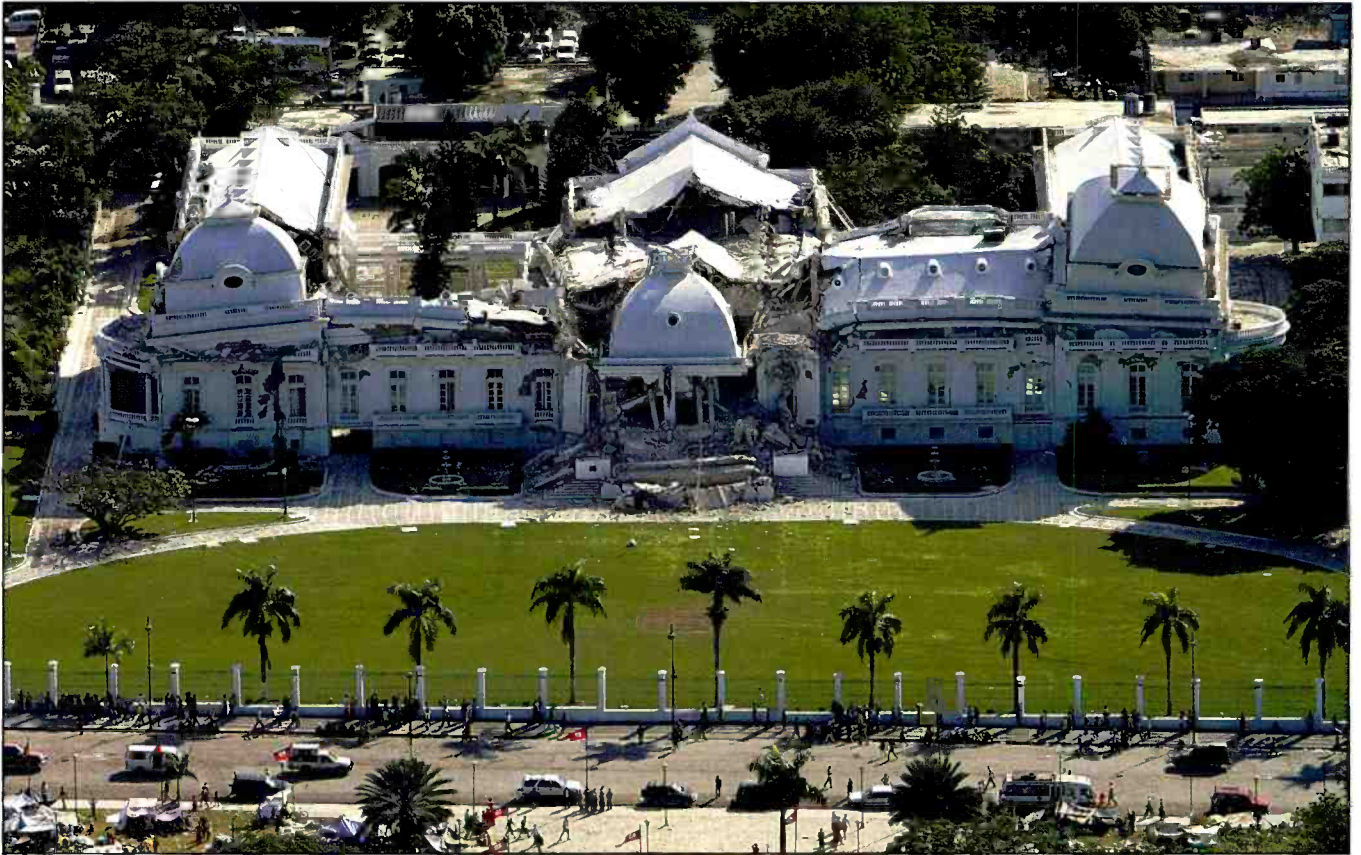
The entire second floor of the Haitian National Palace collapsed onto the first floor after the January 2010 quake. (Public domain photo)
