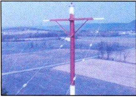
Part of the antenna system at WMLK, Bethel, Pennsylvania. (Thanks Charles Maxant, West Virginia)
