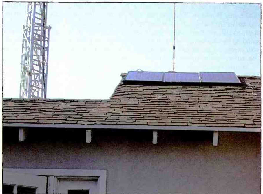
If your area is blessed with sunshine, solar panels are a great source of alternate energy for the whole house. Just remember to regulate solar panel output to levels safe for your radio equipment. Gordo gets 6 amps from these.
