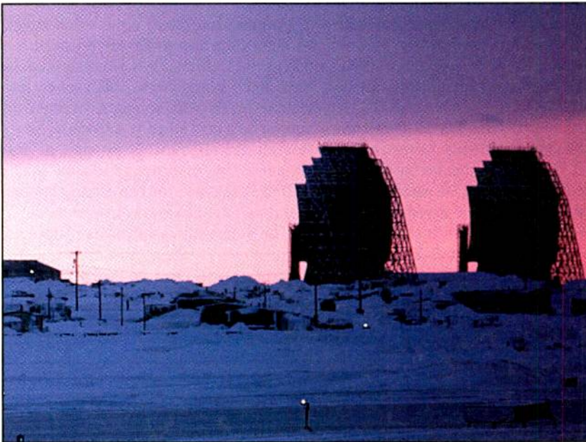
White Alice troposcatter communication antennas designed for troposcatter propagation. The station is one of 30 under U.S. Air Force control. (Photo by Tech. SGT. Donald L. Wetterman, U.S. Air Force)
