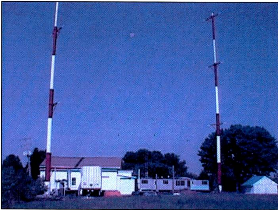
The re-erected antennas at WMLK, which had been downed in a monster ice storm. The transmitter building sits just behind them. (Thanks Charles Maxant, WV)
