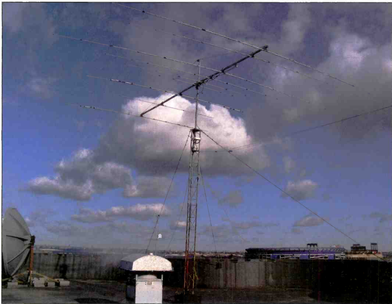
The roof of the Hall of Science, showing the Hall of Science Amateur Radio Club’s (HOSARC) HF antenna, with Shea Stadium in the distance.
