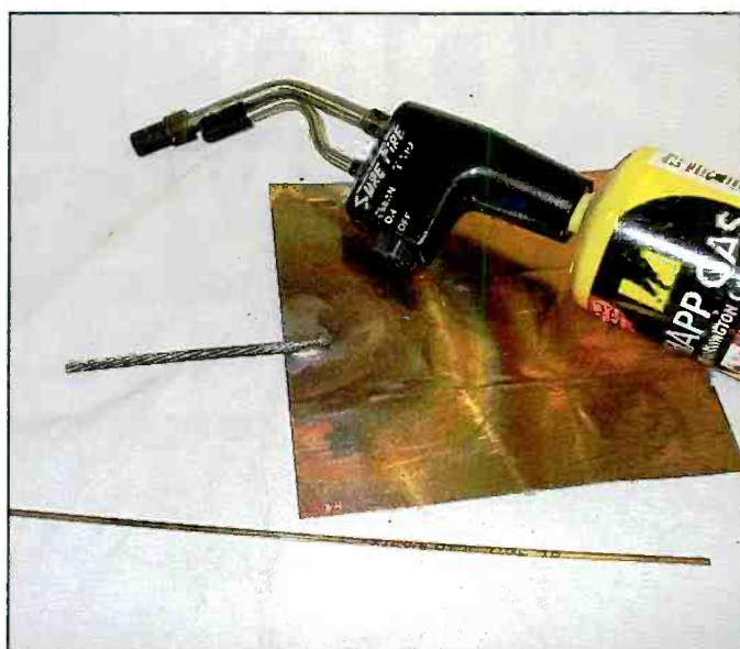
Completed weld. It took only a few drops of the welding rod to make a very secure weld. Note the change in color of the copper. To make the rod flow, the copper needs to be brought up to an almost red color.
