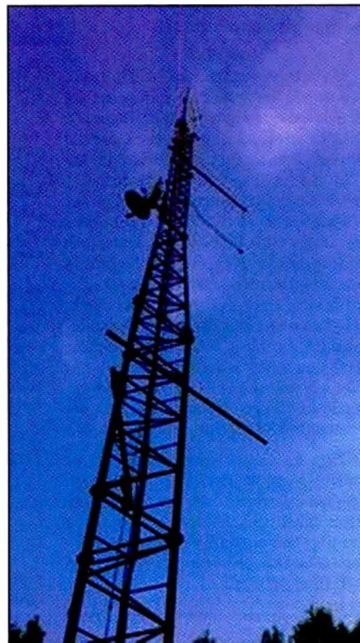
Figure 1. The anti skywave antenna used in the French DRM tests. (Photo from http://drcotedazur.canalblog.com/ )
