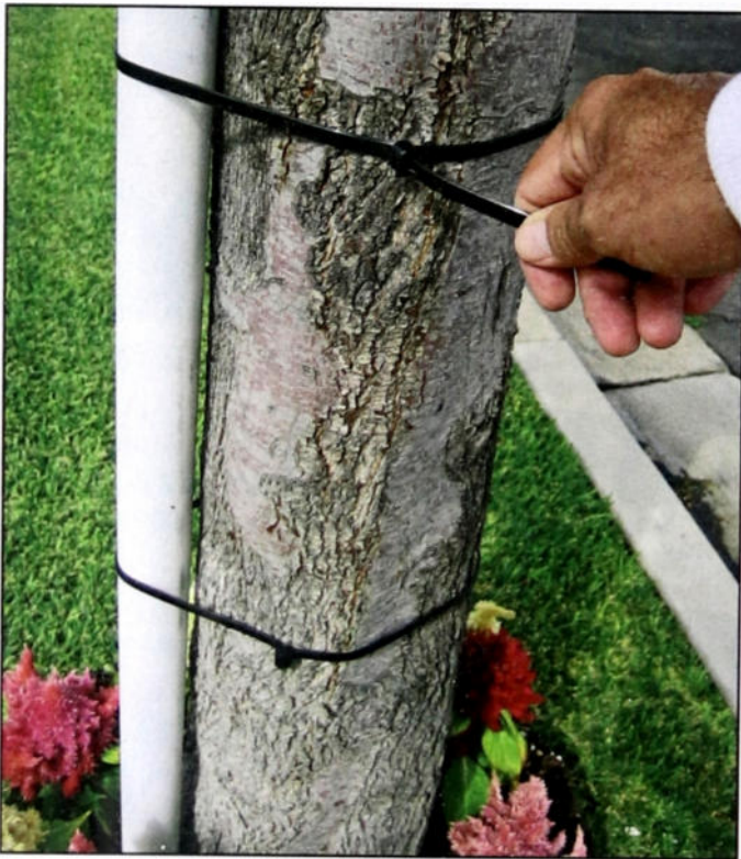
Photo D. Replace all tie-wraps used to secure a mast to a tree periodically, and be sure not to tighten the tie-wrap to the point where it digs into the tree's bark.
