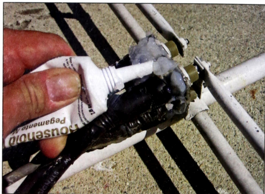
Photo C. Silicone sealant helps protect connectors located in tight areas where effective tape winding isn't possible.
