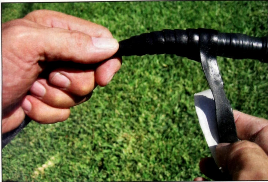
Photo B. Covering a coaxial cable mid-span splice with a sealing compound like COAX-SEAL ensures a watertight connection.
