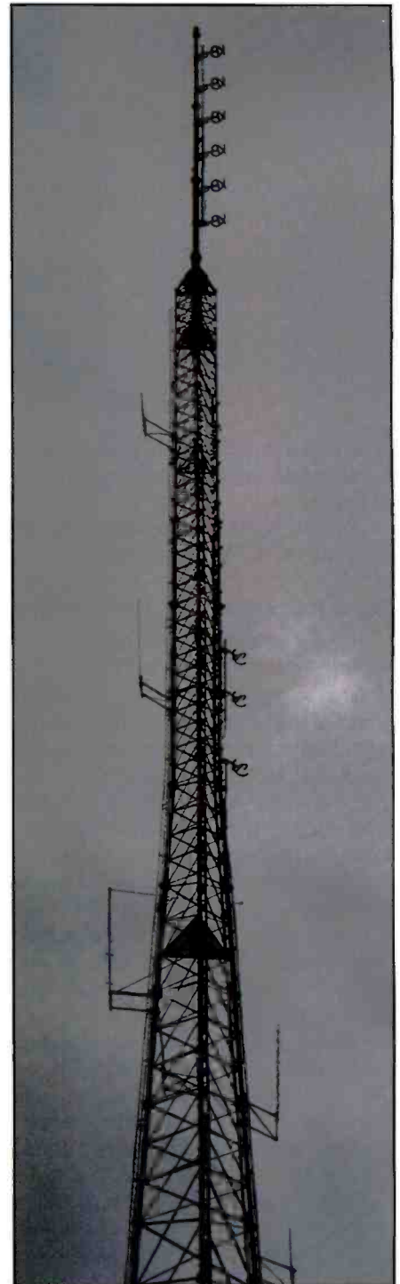
In many metropolitan areas, competition for tower space is at a premium, not to mention high-rise buildings to put them on. This antenna system outside St. Louis is carrying four or five systems, plus a radio station and, lower down, a cellular system.
