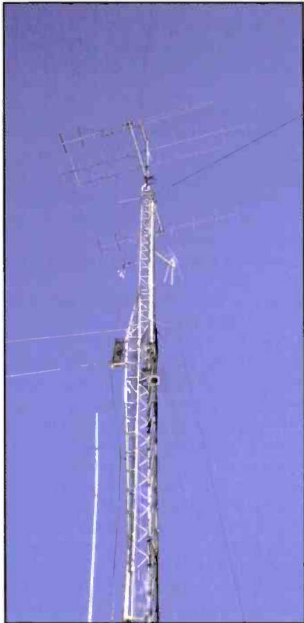
Here's a 65-foot recycled Rohn 25G tower supporting VHF and UHF ham antennas.
