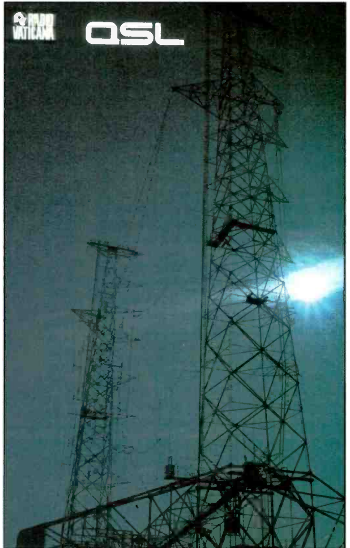
One of the rotating towers at Vatican Radio's Galeria site.
