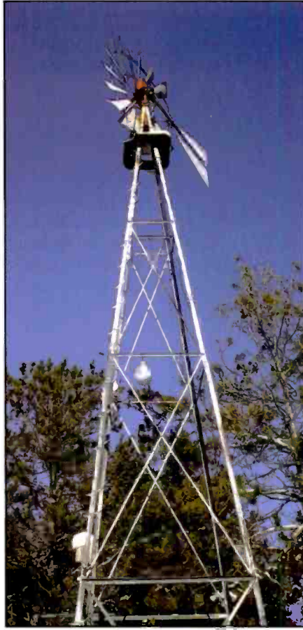
An old farm water pump windmill tower recycled into holding up the ends of ham wire antennas.
