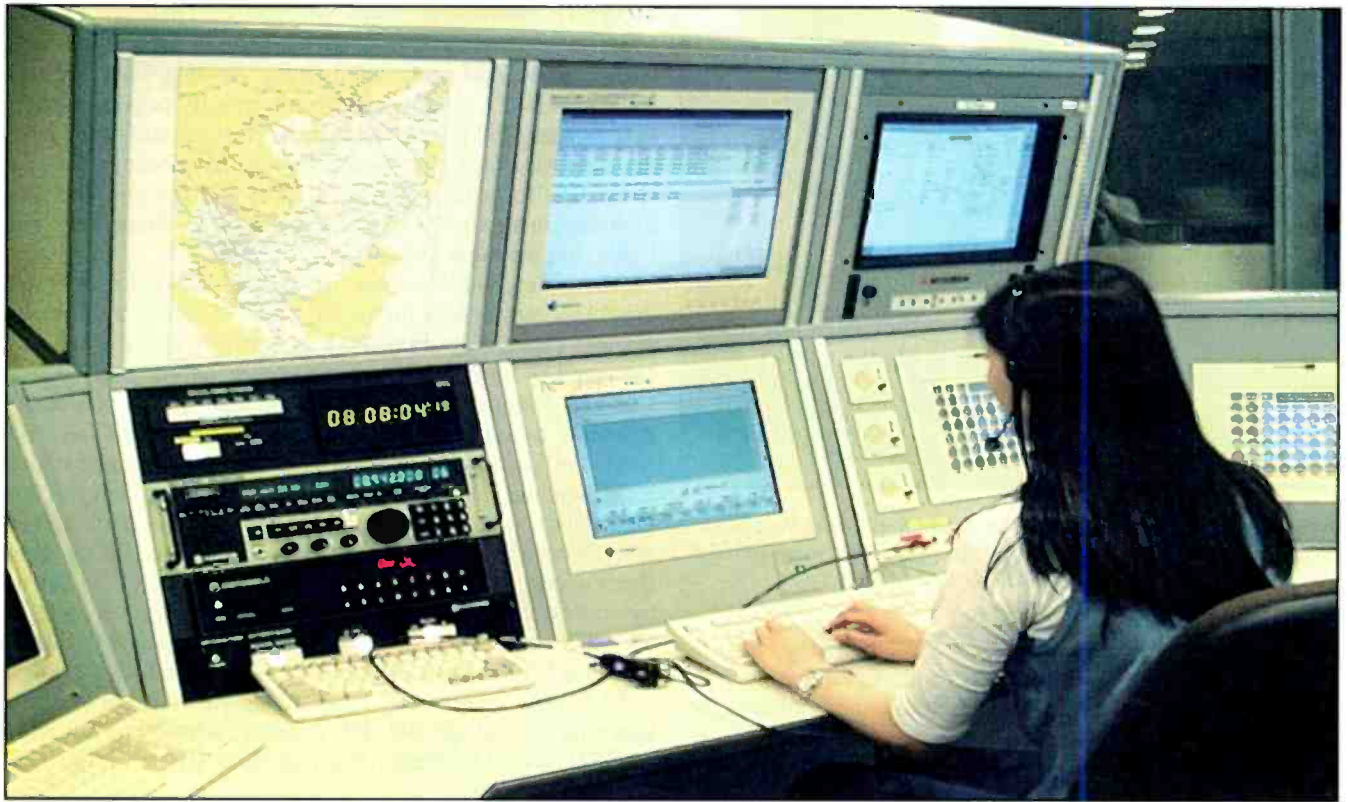
Photo B. The HF radio console at the Hong Kong HF aeronautical station. (Courtesy Hong Kong Civil Aviation Department)
