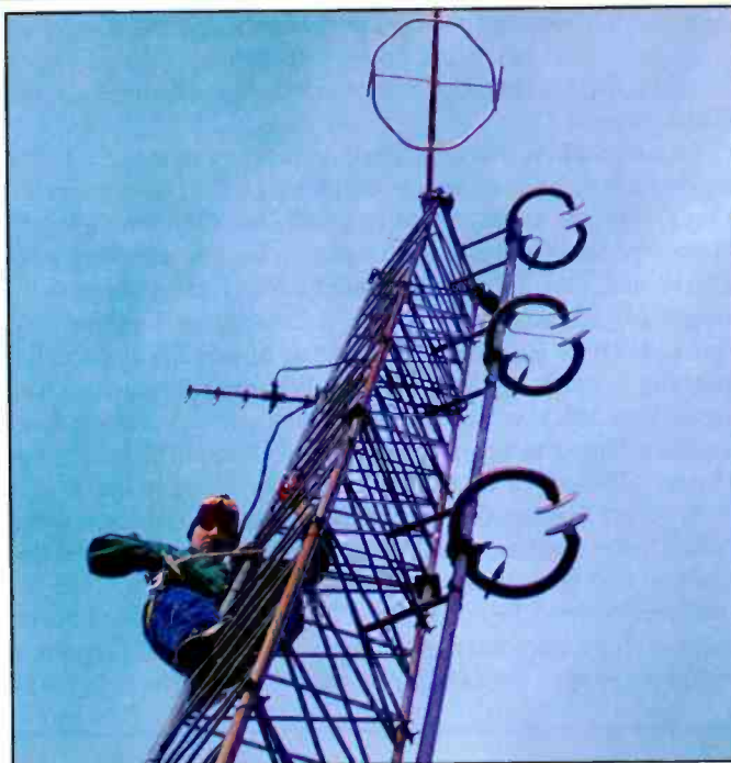
It's not all studio work. Josh Jones, North Dakota State University student and KNDS chief engineer, goes tower climbing for the installation of the station's single bay ERI antenna.
