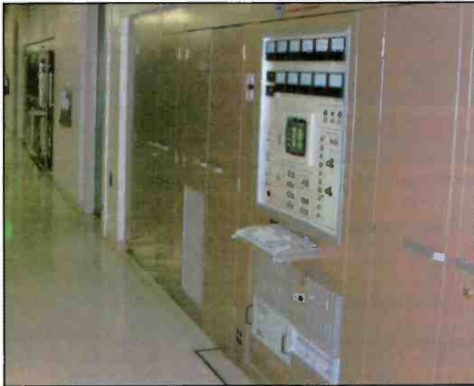
One of the four 500-kW transmitters housed in WEWN's transmitter hall at Vandiver, Alabama. (Thanks Charles Maxant)
