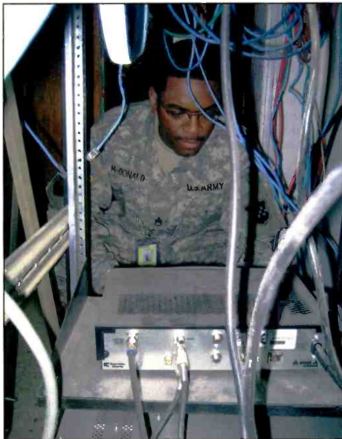
Staff Sgt. Christopher McDonald, chief of technical engineering for AFN-Iraq, inspects the transmitter that his team recently installed on the top floor of the U.S. Embassy in Iraq. The transmitter greatly improved radio reception in Baghdad's International Zone. (All photos by Maj. Gary Sheftick)
