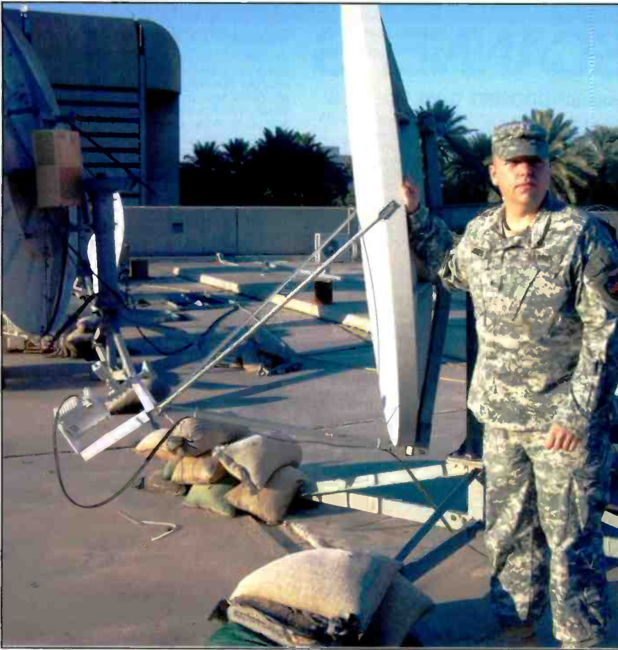
Sgt. Matthew Jones points out the microwave dish that sends the Freedom Radio signal from the roof of the AFN-Iraq studios to Mannheim, Germany. From Germany the signal is relayed to forward operating bases in Iraq and Kuwait.
