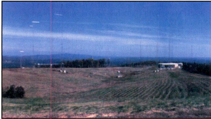
The building on the right at the WEWN site houses four 500-kW transmitters! (Thanks Charles Maxant, WV)
