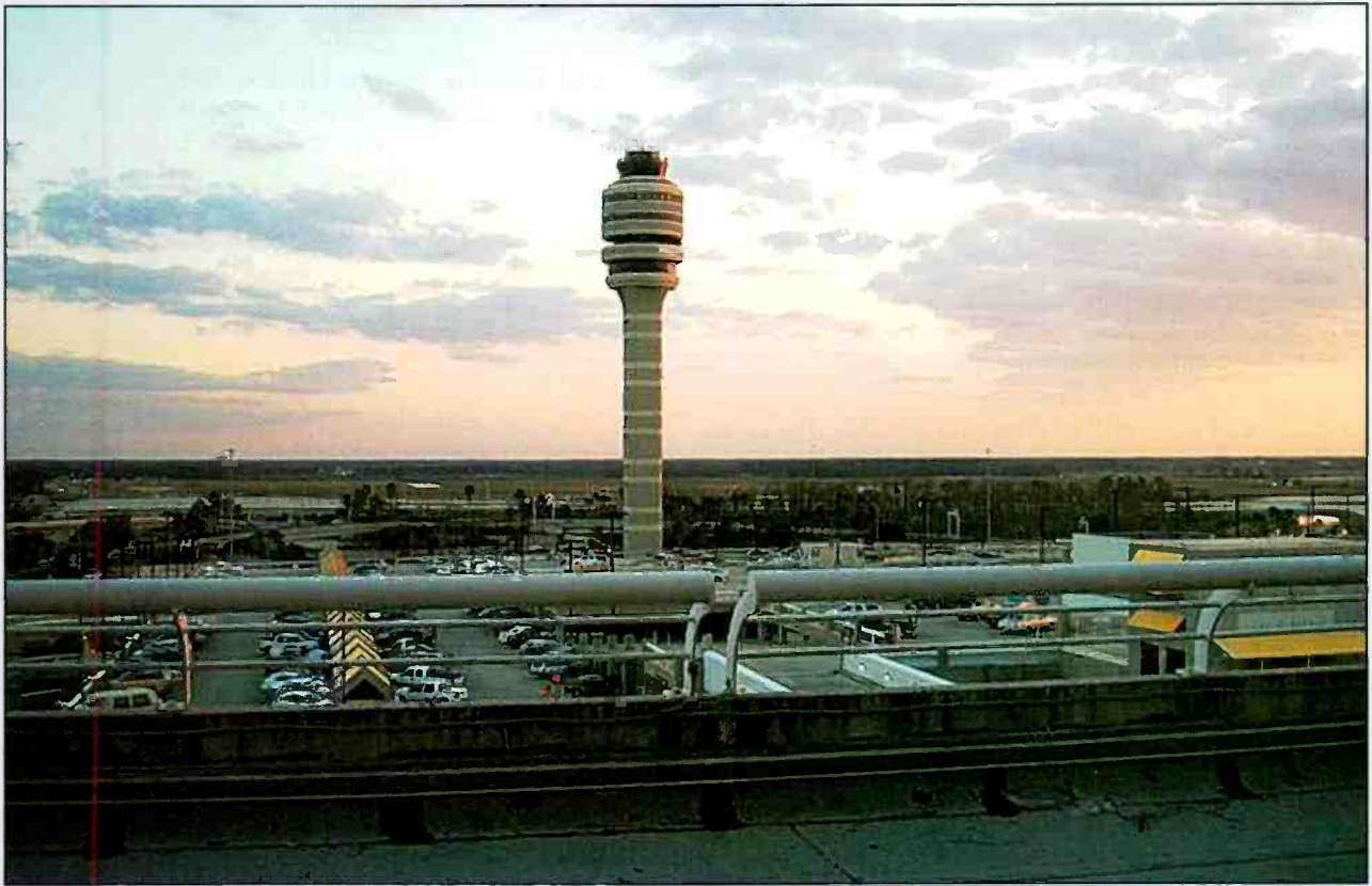
Control tower at the Orlando Airport.
