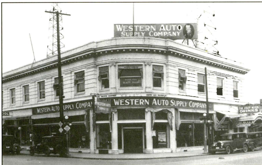
Signs on downtown Medford's Sparta Building hawked everything from Western Auto wares to "eats, pool, beauty shop" and "drinks." Nowhere in this circa-1929 scene, however, were the call letters KMED, but those towers on the structure's roof shout "radio!" The towers were supposed to hold windmills to help pump water on a couple of Oregon farms, but were bought from the local Grange before they could get enlisted for such bucolic endeavors. Strung with copper wires, they instead served to wing KMED's 50-watt signal to Medford area listeners.
