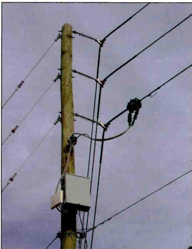
Here's a pole-mounted "injector." All the pole-mounted boxes look the same: injector, repeater, and extractor.
