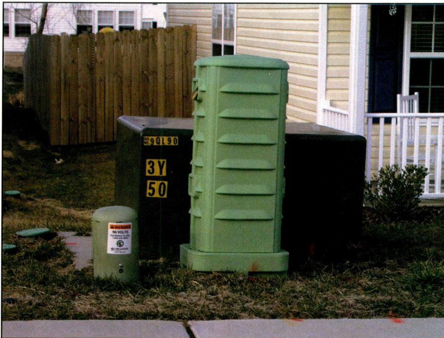
This pedestal, in North Carolina, is in the tall, lighter green box with its cover on.
