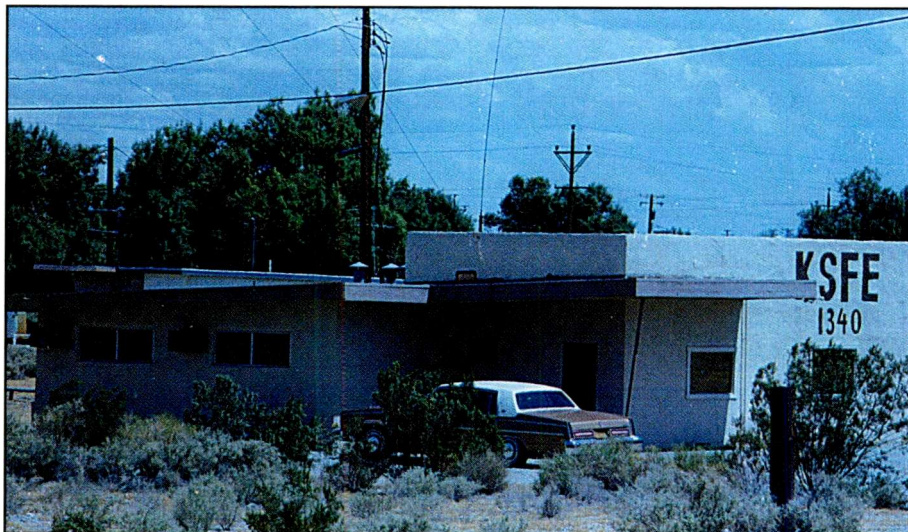
Built in 1948, this building was home to two very different KSFE stations. Notice that the windows are all boarded up, presumably for keeping drifters and stranded motorists along the nearby interstate highway from trying to break in or to noisily summon the DJ's attention. (Courtesy of Jan Lowry, 1982)
