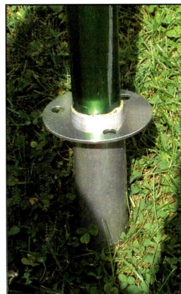
Slip the guy ring over the tube prior to mounting the antenna.
