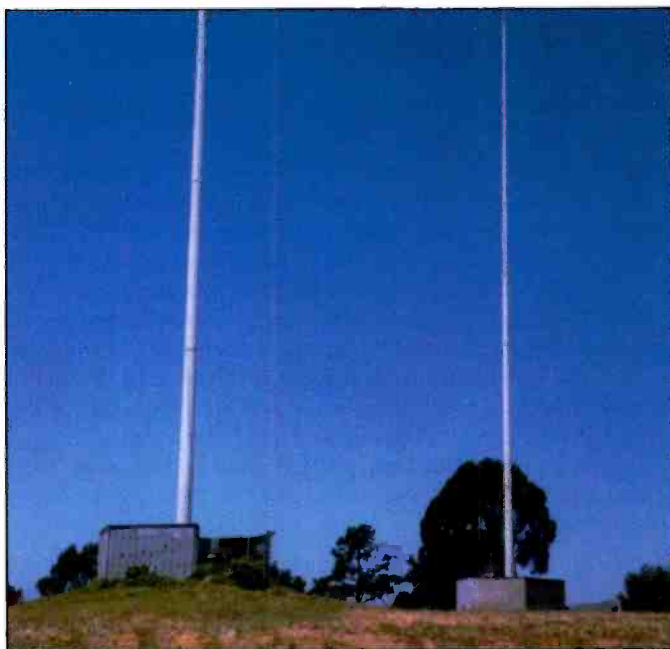
Thought I'd throw in a shot of two of the four tubular towers of KMBY 1540 kHz in Capitola, California. Jan Lowry snapped the picture and reports the "pole" towers were painted white and were fed by a transmitter in a small metal building located off State Route 1, between Aptos and Capitola. Apparently KMBY has been silent since October 1995. Jan couldn't detect any local signal when he tuned his vehicle's radio to 1540.
