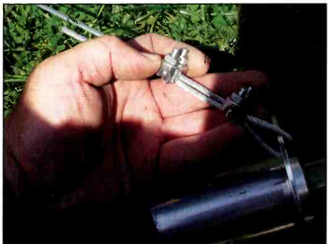
Three sections of heavy-duty guy wire were used to keep the SteppIR BigIR antenna secure in high winds.
