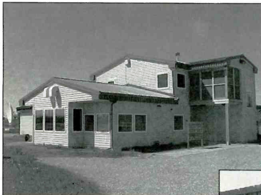
Northway FSS facility.
