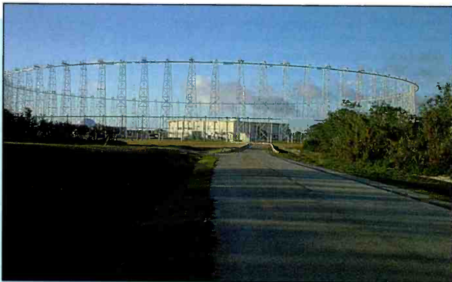
Before the advent of satellite-based navigation the U.S. Navy operated an extensive HF direction finding network. PopComm reader, Fred Muller took this picture in May 2000. It shows the Wullenweber antenna located at the Naval Computer and Telecommunications Station on Guam. The station is now decommissioned and has been all but abandoned.
