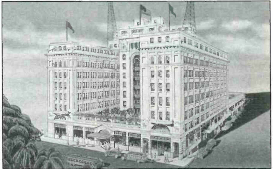
Another view of KFSD's leaning towers.
