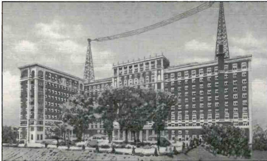
WSB, long one of America's best known stations, had its antenna atop Atlanta's prestigious Atlanta Biltmore Hotel.
