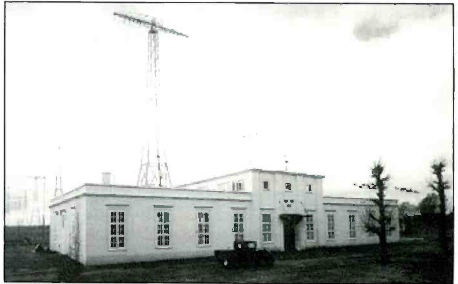
Grimeton transmitter site in Sweden with LF vertical antenna pointing at the U.S.
