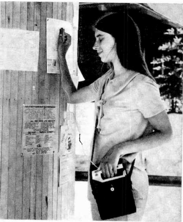
Shari Gabrielson, Berkeley High School student, reads bulletin board with an Optacon reading machine developed at Stanford Univ. While scanning with probe in right hand, her left hand makes contact with an array of tiny tactile stimulators which form outline of each scanned letter. Single finger tip can be employed to read the letters.
