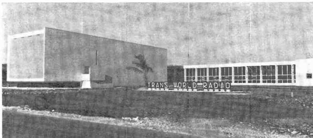
The new studio and office building of Trans World Radio , Bonaire, Netherlands Antilles, is one of the most advanced of its type in the world. It is unique in that it has acoustical floating walls, reverberation control, absorption panels and sound proofing. The gigantic antenna complex was erected several years ago.
