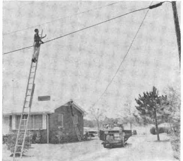
Cable can be run underground or on poles. Space on existing poles is rented for about $2.50 per pole, annually, plus insurance. Experienced crew can string up to 14 miles a day.
