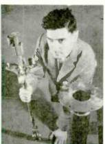
Hughes' maser microwave amplif er has ruby and magnet at bottom. Lnt is installed in coolant container (above, right) to supercool ruby near absolute zero.
