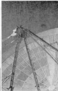
NASA parabolic artenna catches fleeting signals from space; they're amplified by supercooled ruby maser mounted in front.
