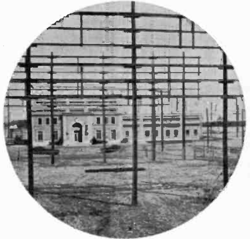
Ship's position is plotted (inset) and optimum antenna, transmitter, are chosen for communications by shore-based technicians. Transmitting station at Lawrenceville, N.J. (top) contains banks of transmitters. Rhombic antennas (above) direct calls toward Europe, Africa, and South America from New Jersey.
