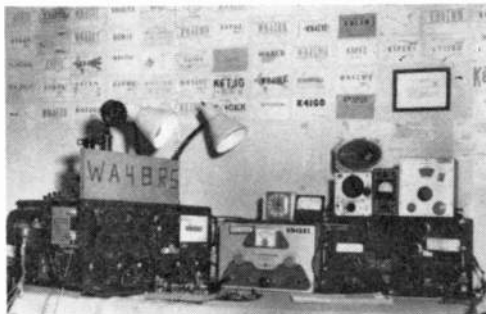
Paul Folmsbee, WA4BRS, Laurinburg, N.C., sticks to 75-meter phone and 80-meter c.w. with his Heathkit DX-40 transmitter and BC-342 receiver. He also uses a war-surplus ART-13 2000-watt transmitter.
