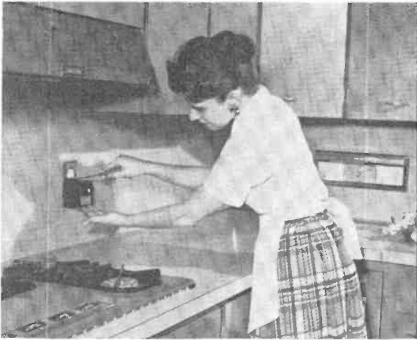
Fig. 2. Black box receiver (right) plugs into a.c. outlet and can be installed in a few minutes. Flange on receiver is designed to accept face-plate screw of receptacle and holds unit securely in place.
