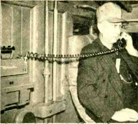
In the caboose of this train, a Motorola walkie-talkie is used in lieu of a regular, high-powered mobile communication set.
