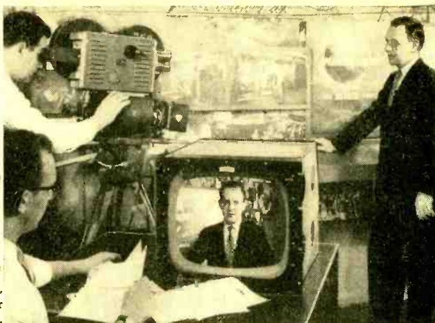
Mounted atop a 35 mm. movie camera, the new "Tel-Eye" provides director with same view recorded by camera.
