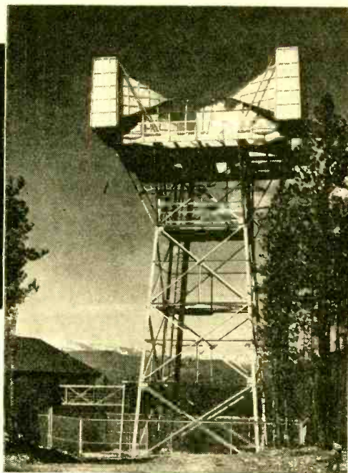
One of the stations on the Bell System's radio-relay route between New York and San Francisco.
